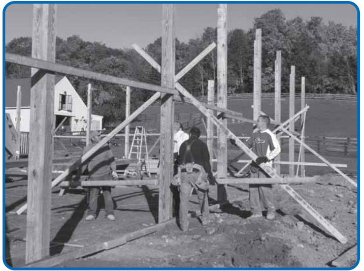
Contractors erect and stabilize the framing for the covered outdoor arena.
